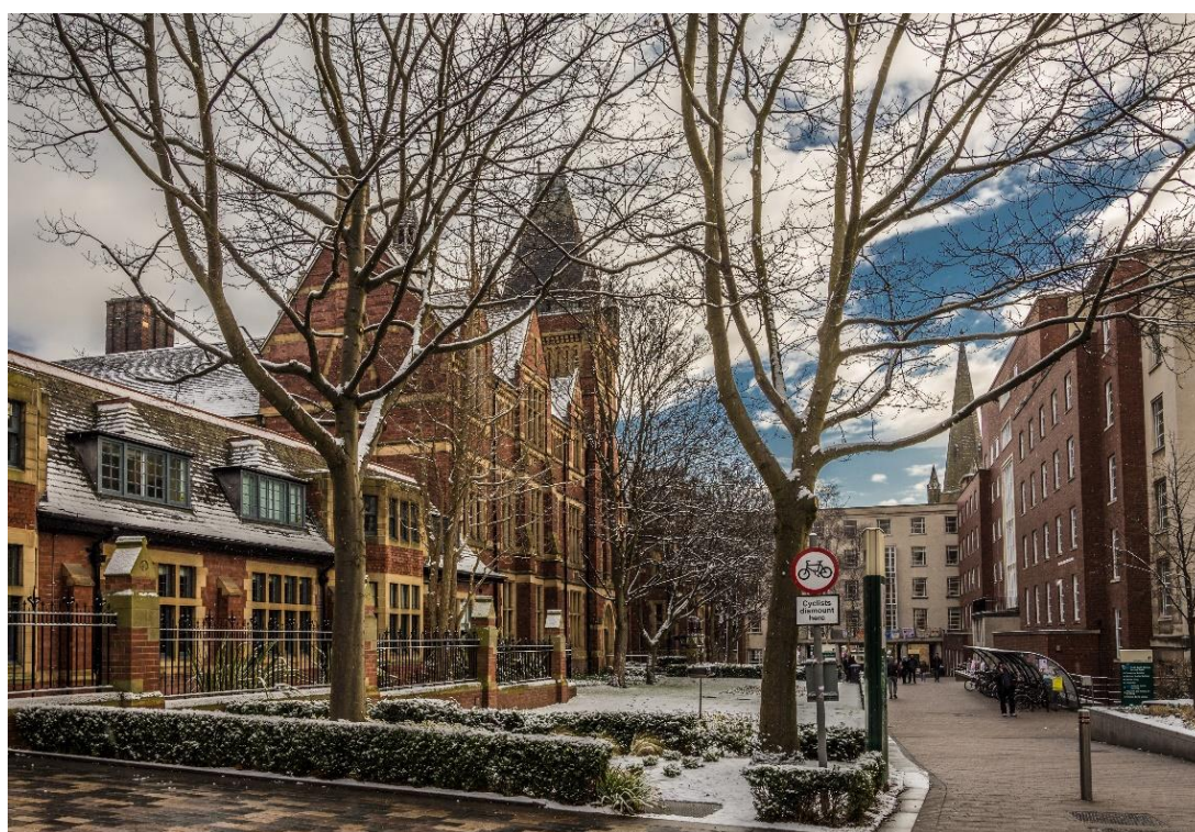
The red brick building on the right is the Michael Sadler Building. The white porched door gives direct entrance to the Rupert Beckett Lecture Theatre, down one flight of stairs.
